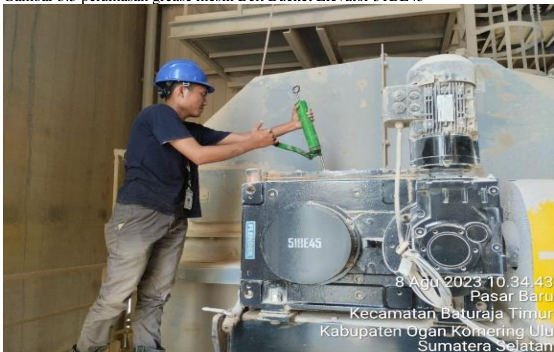
Gambar 3.5 pelumasan grease mesin Belt Bucket Elevator 51BE45
